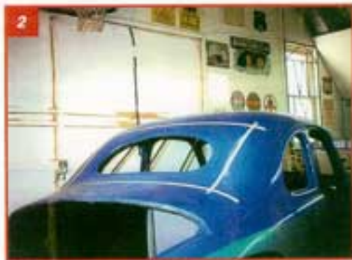
Photo 2 displays the inside of the shop where we stripped the glass and started to brace the inner structure with 1" water pipe. We ran the braces side-to-side and front-to-back. The structure was
